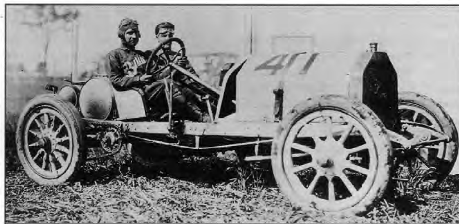
Bob Burman at the wheel of a Marquette-Buick in 1910. Photo is rare in that "Buick" script is shown on the radiator. The word "Roadster" appears under the "Buick" script. This was a part of Buick's attempt to hide the fact that the cars were not stock. (Courtesy of Greg Fauth)
