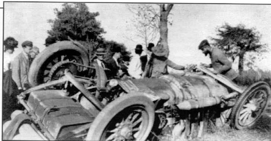
Buick "stealth" photo at 1908 Savannah Grand Prize. Walter Marr—peering over front end of wrecked Benz—learns how Benz designed the suspension in its highly successful ohv race cars.
